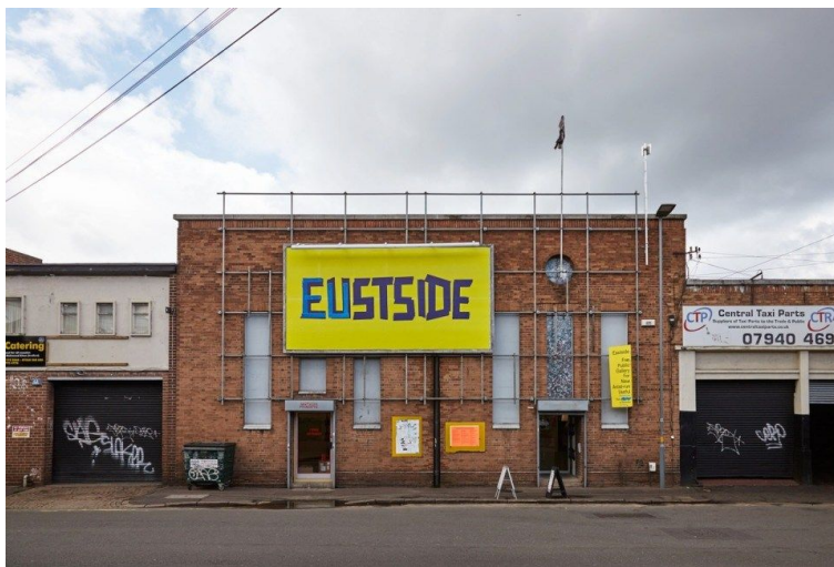
Kathrin Bohm, EUStside 2016, Eastside Projects Facade, billboard poster on: Céline Condorelli & Gavin Wade, Scaffold as declaration of altered conditions 2008, Temporary External and Internal Façades, scaffold tubes, scaffold fixings, scaffold boards, Billboard hoardings constructed of timber, paint, electrical fittings for outdoor lighting. 5m x 12m x 0.3m and 5m x 12m x 10m. Photo by Stuart Whipps.
